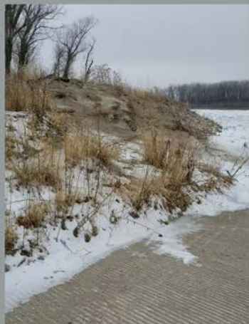
Site 4: Boat Ramp - Southerly Side
