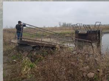
Site 1: Stop Log Structure
