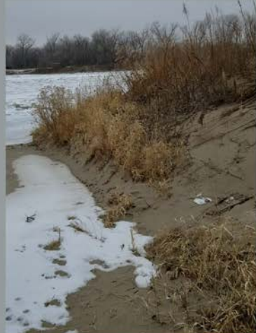
Site 4: Boat Ramp - Northerly Side
